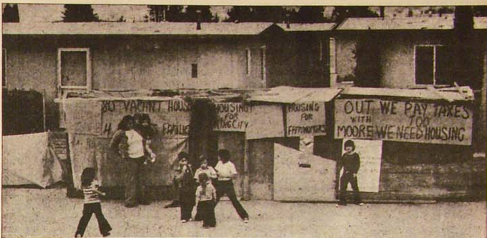
Plywood shacks built by Chicano families who were evicted from a state-run housing camp.
